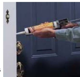
Caulk around the doorway to keep out drafts.
